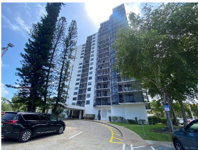
Photograph B1: Overview
